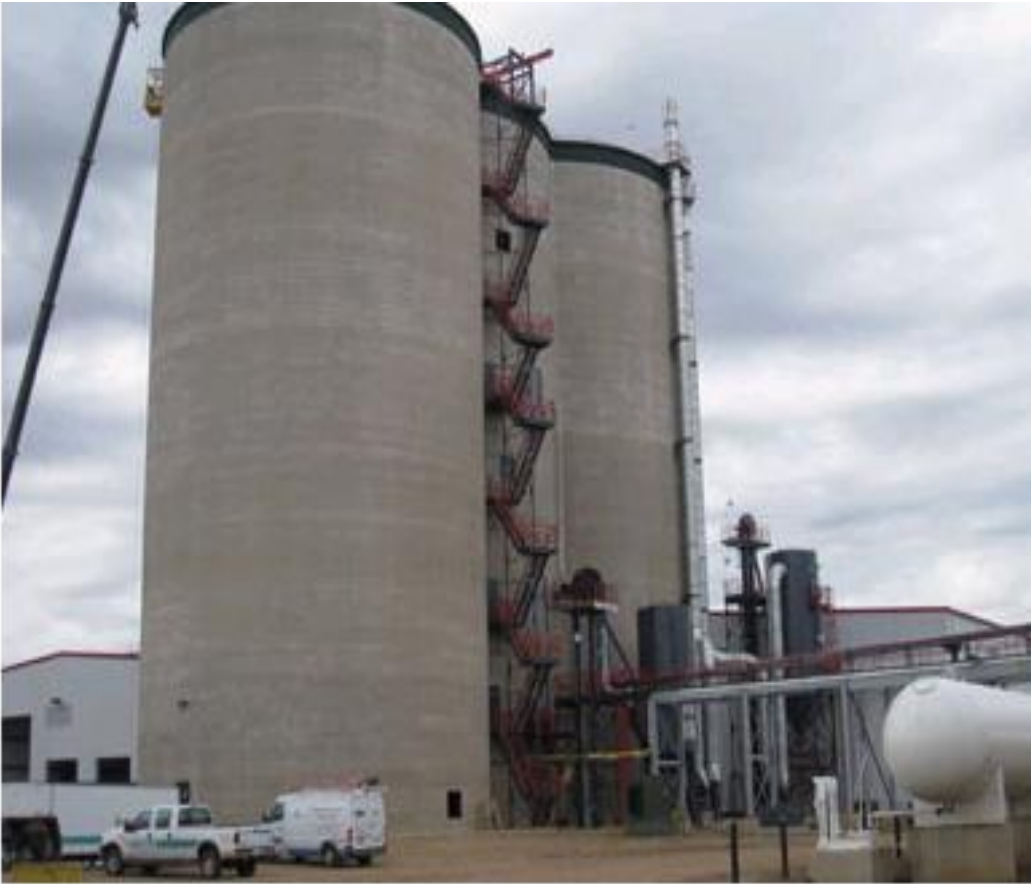
Poured concrete Silos (2+)
