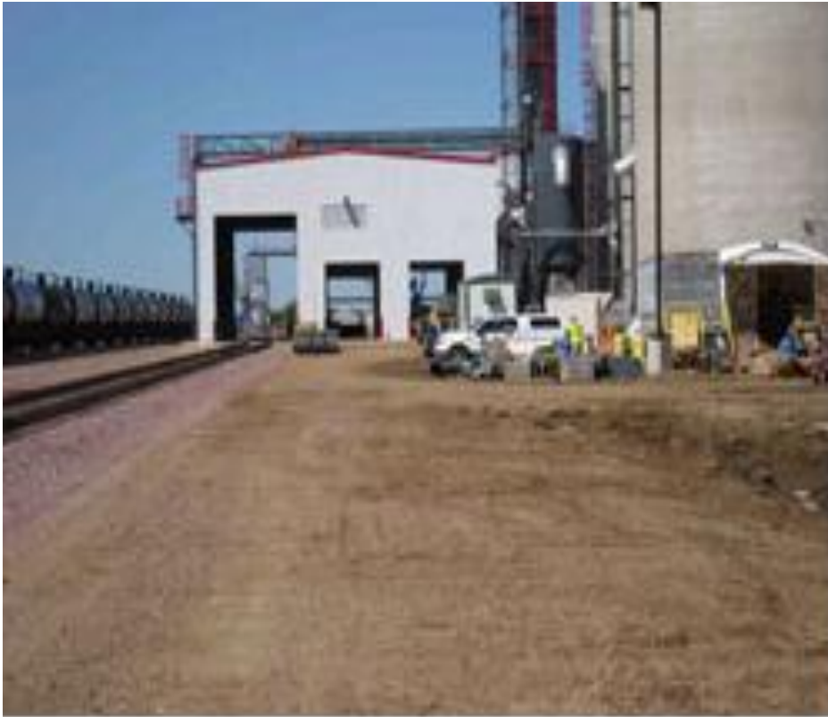
Grain Receiving Bldg w/rail spur
